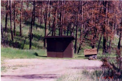
Figure 3.3: Pump building and cap. (Source: QE|A 2003, Roll7-16)
