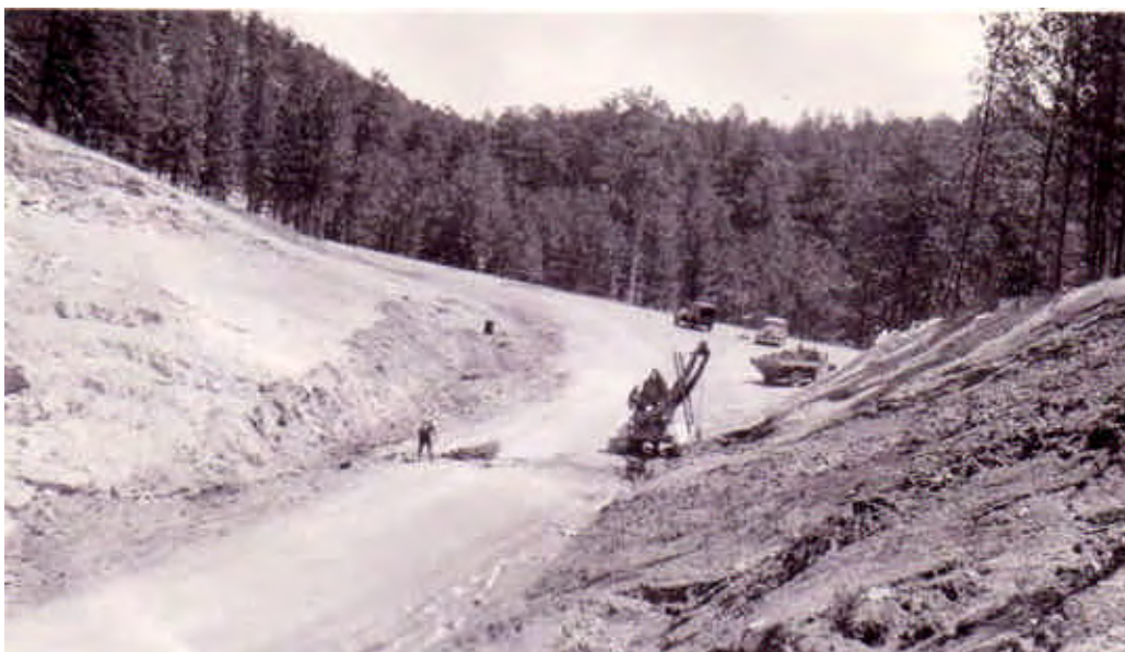
Figure 2.19: Highway 16 Construction, 1937 (Source: JECA 2898)
