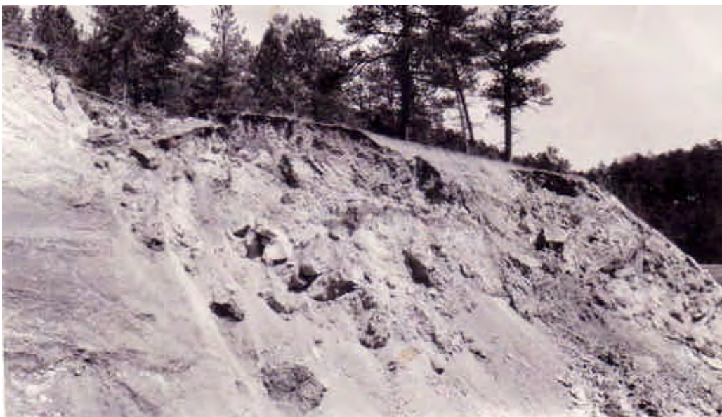
Figure 2.17: 1933 “landslide across from entrance road” (JECA 2801)
