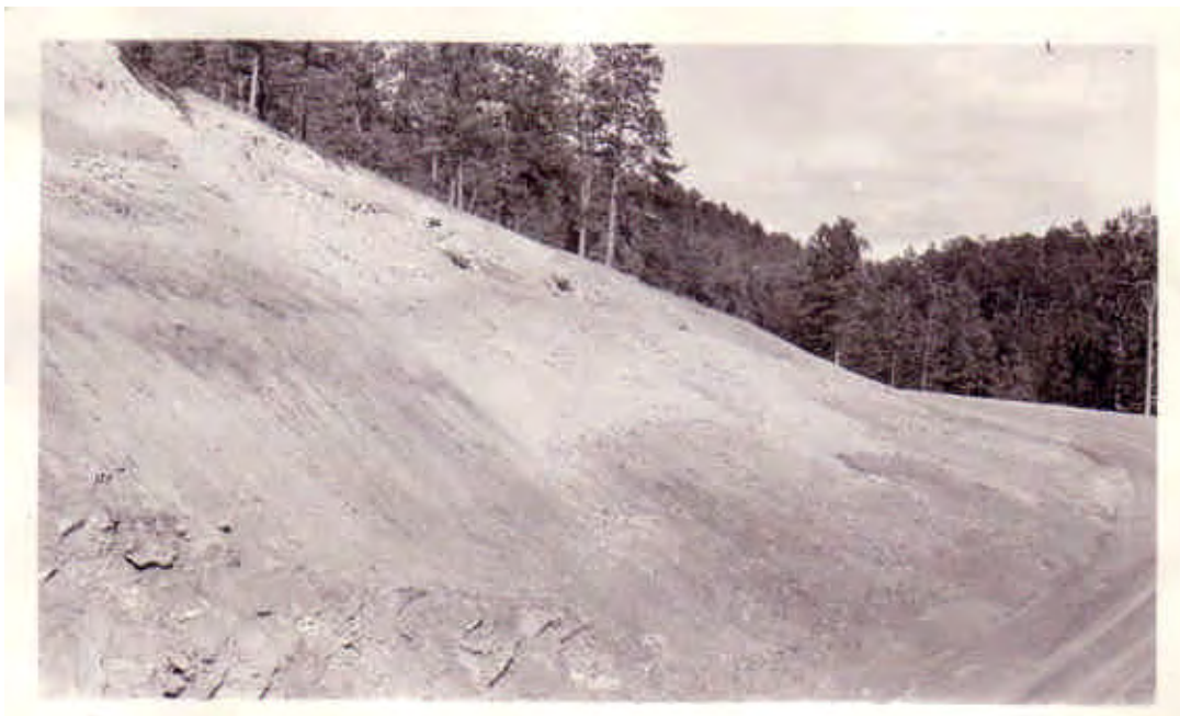
Figure 2.18: Slope graded for new road, 1933 (JECA 2803)
