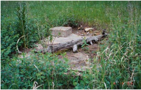
Figure 3.47: Concrete foundation, remnant of former structure in Hell Canyon. (Source: QE|A 2003, Roll 1-23)
