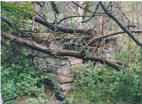
Figure 3.48: Remnants of fireplace in Hell Canyon. (Source: QE|A 2003, Roll 1-22)
