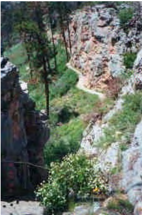
Figure 3.37: View of Lower trail and area of CCC retaining wall from stone stairway (Source: QE|A 2003, Roll5-1)
