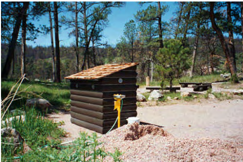
Figure 3.7: Lantern Storage and Eyewash Station (source: QE|A 2003, Roll2, AA007A)
