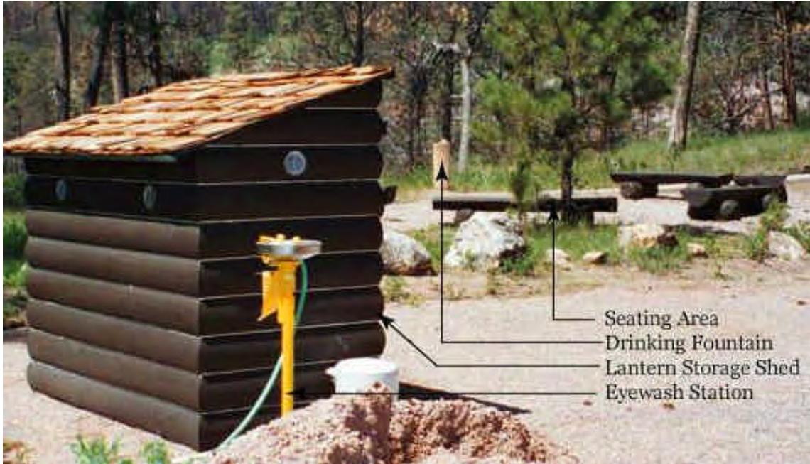
Figure 3.54: Lantern storage shed, eyewash station, circular seating area, and drinking fountain. (Source: QE|A 2003, Roll 2-7)
