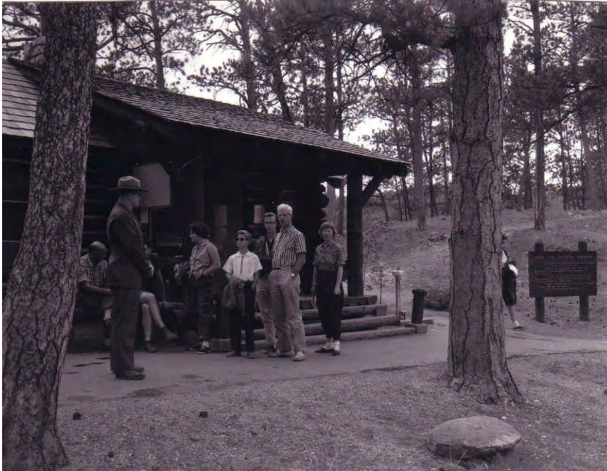
Figure 59: Ranger Cabin, drinking fountain, sign, and bench, 1961 (Source: JECA 2082)
