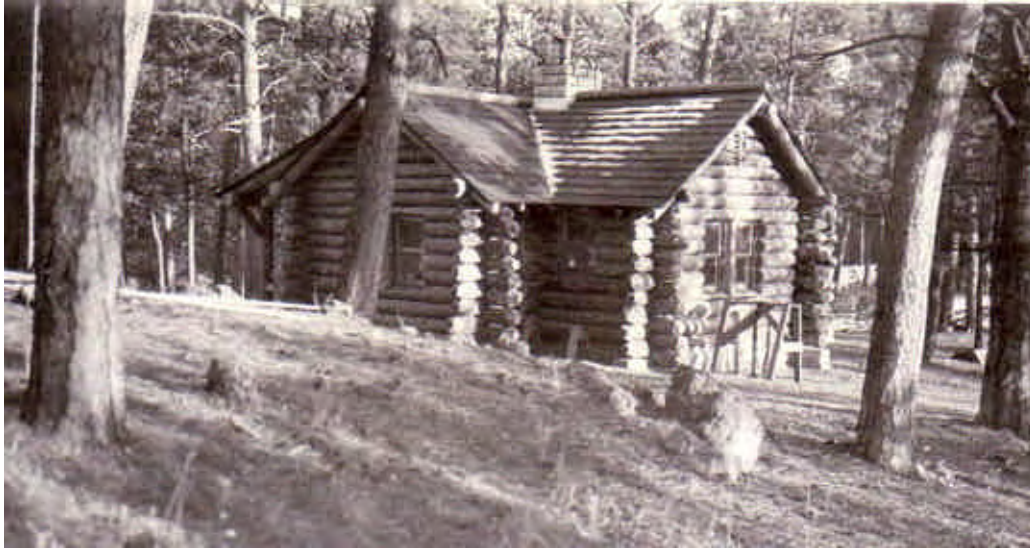
Figure 2.34: Ranger Cabin, north and west sides, 1935 (Source: JECA 2628 and Rugged Charm: Ranger Cabin Historic Structure Report , 1999, Figure 6)
